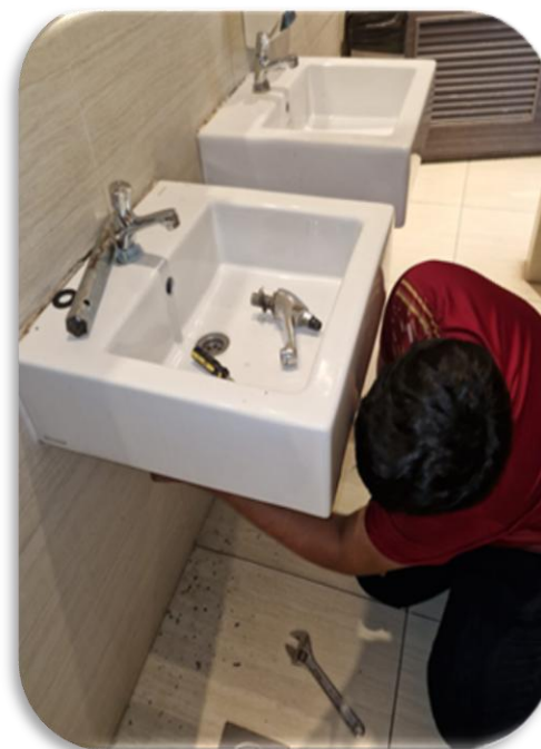
Replacing Water Faucet @ HomeTeam NS
