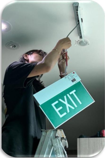
Installing Emergency Exit Light @ Civil Service Club
