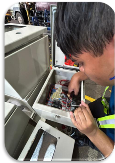
Checking Electrical Control Circuit @ Wong Fong Engineering Works (1988) Pte Ltd
